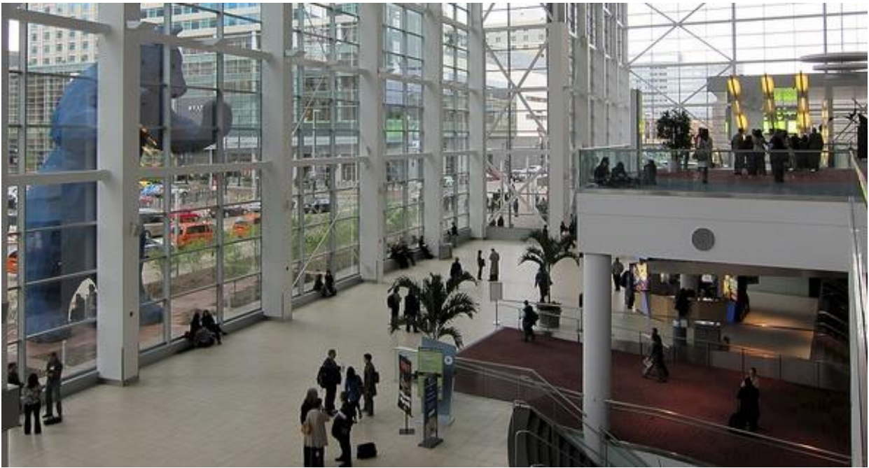
Main ramp at center of lobby exceeds 10%
